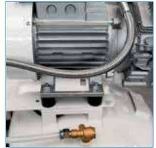
Pump unit mounted on anti-vibration devices
