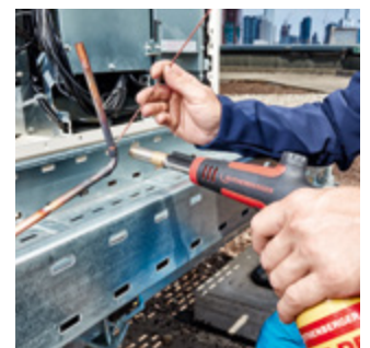
Brazing in refrigeration / air-conditioning technology
