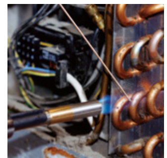
Brazing in refrigeration / air-conditioning technology
