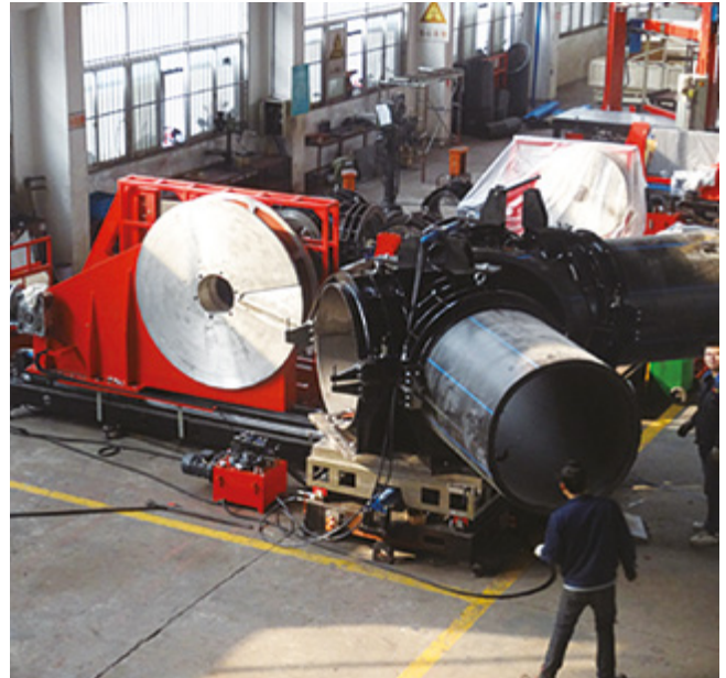
Production of a Y-piece on a workshop machine
